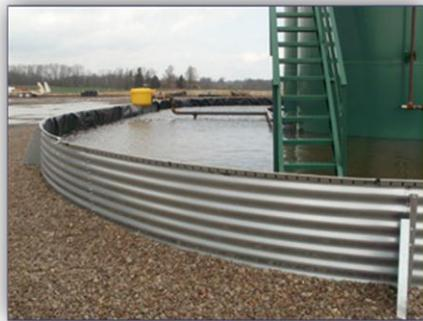
*“Rain water will fill up containment structures, reducing the amount of hazardous chemicals they will hold in case of a spill. The R.S.S. will prevent this from happening.”*
